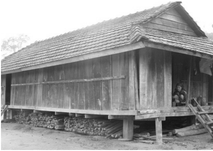
Figure 14: Housing style. Photo by SPERI, October 2014
